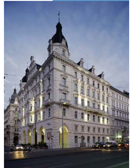
Buchart-Horn is providing Project Management services for the renewal and renovation of the facade of the historic U.S. Consulate Building in Vienna, Austria.
