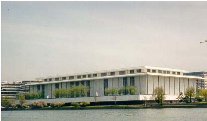
The John F. Kennedy Center for the Performing Arts, Washington DC CPM scheduling and Cost Estimating Services
