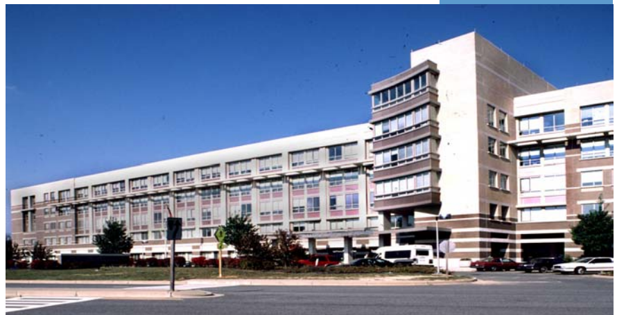
Performed leak detection studies in Naval Air HQ building.
