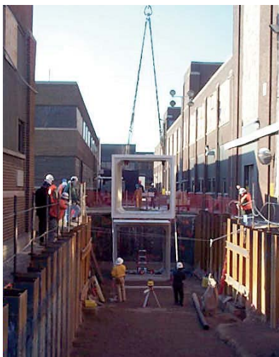
Shaw safely completes Linde site utility tunnel replacement.
