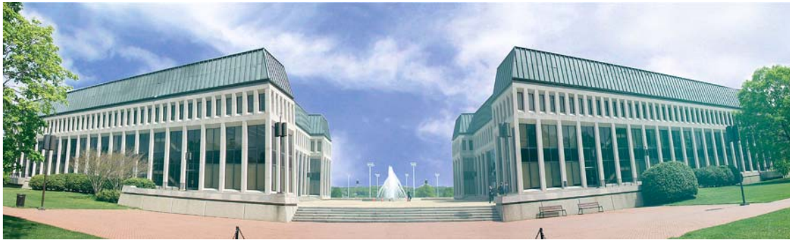
HOK was selected by the U.S. Navy Engineering Field Activity Chesapeake to renovate this 270,000 GSF academic complex on the historical quadrangle of the U.S. Naval Academy.
