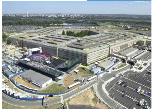
The Phoenix Project encompassed over 400,000 SF of existing building that had to first be entirely demolished due to the extent of the damage.
