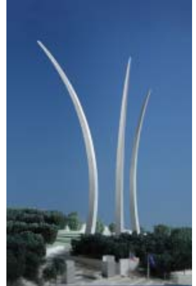
US Air Force Memorial - ECS has provided geotechnical and environmental consulting services during the design phase of the new Air Force memorial project in Arlington.
