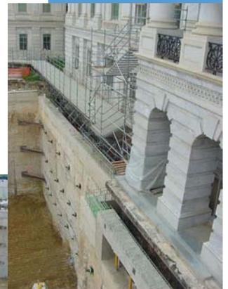
More than 500 truckloads of material continue to be removed from the site each day and the perimeter slurry wall, 2,080 linear feet, is complete.
