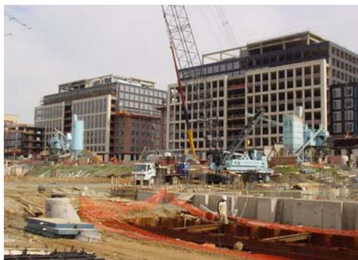
*ECS is currently operating an on-site laboratory and is providing full testing and inspection services during construction, including earthwork, mat and pile foundation construction, waterproofing, fluid concrete placement including certification and periodic inspection of three site concrete batch plants, roofing, structural steel, and structural precast for this 3.4 million square foot complex.*
