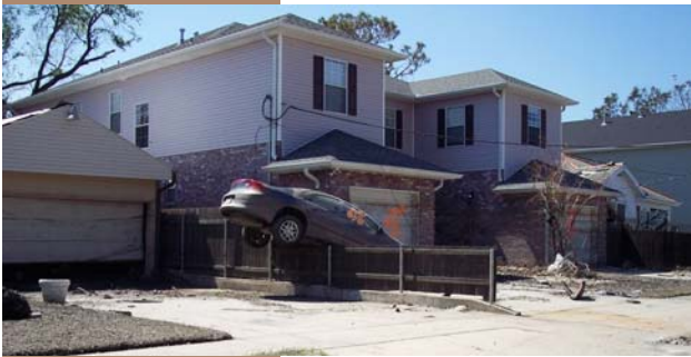
Hurricane Katrina flood waters re-parked cars in Orleans Parish.
