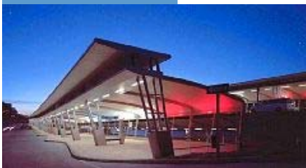
Pentagon Metro Entrance Facility
